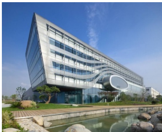
Gambar 2. Envision Energy Headquarters (Sumber: aecom.com )
